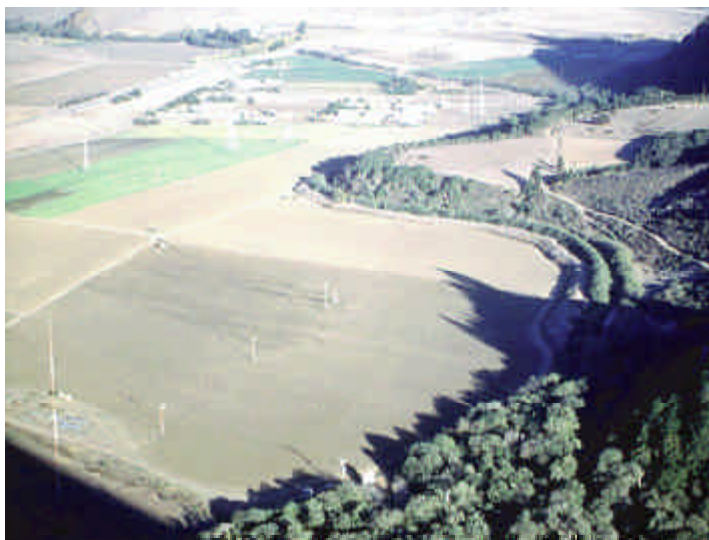
1986 pre-project: Riparian forest eliminated; channel constricted by levee
